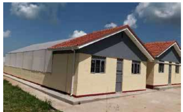
Figure 7: Some of the renovated research infrastructure at NaSARRI
